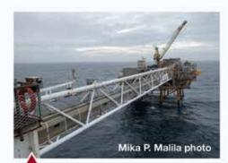
Study used observations from Ekofisk B oil and gas platform in the central North Sea. Lasers in the footbridge measure wave height, timing and distance length between wave crests.
