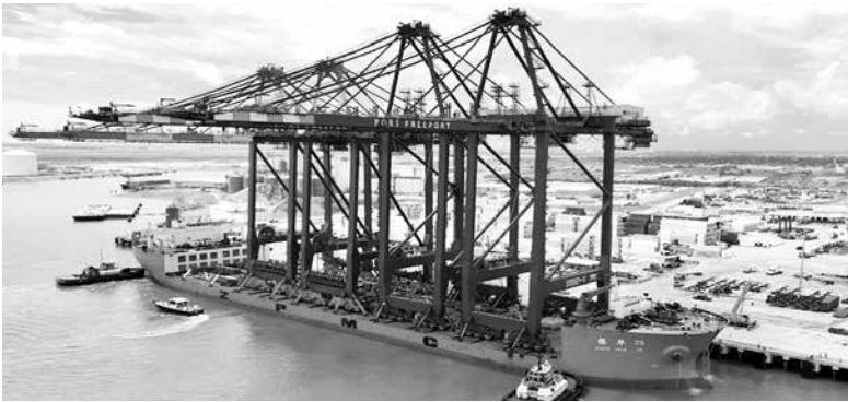
Two state-of-the-art Super Post-Panamax Gantry Cranes were delivered aboard a heavy-lift vessel, arriving at Port Freeport's Velasco Container Terminal.
